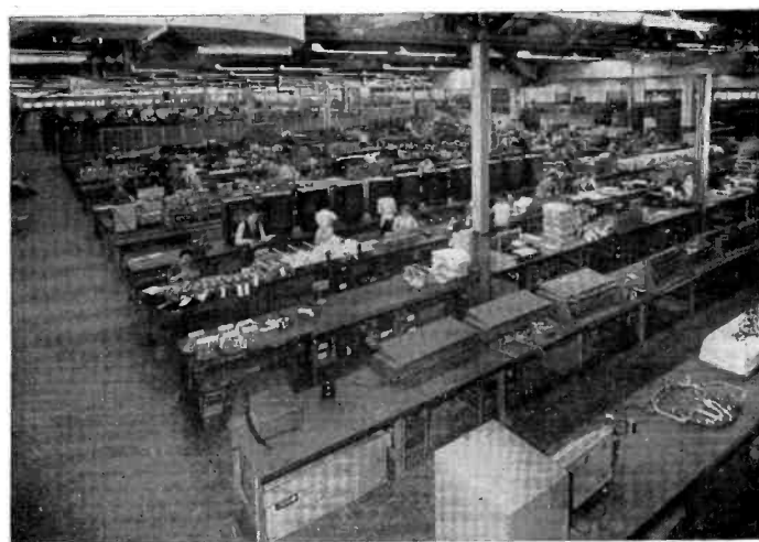
Interior of Transmitter building at Electronics Park.
